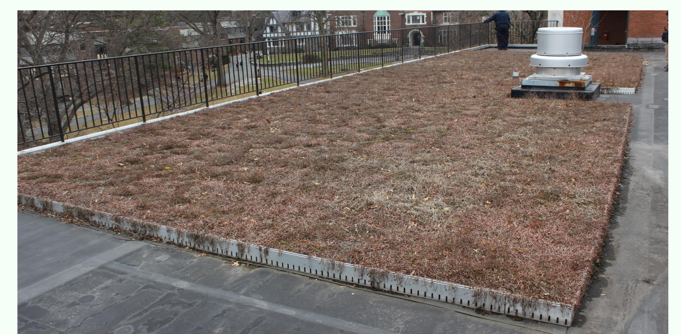
Current state of Taylor Green Roof - March 2016
